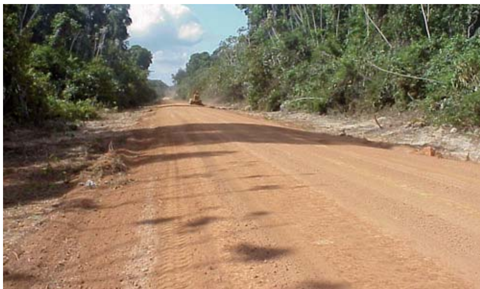
A section of the Guyana/Brazil road. To be opened mid 2009.
